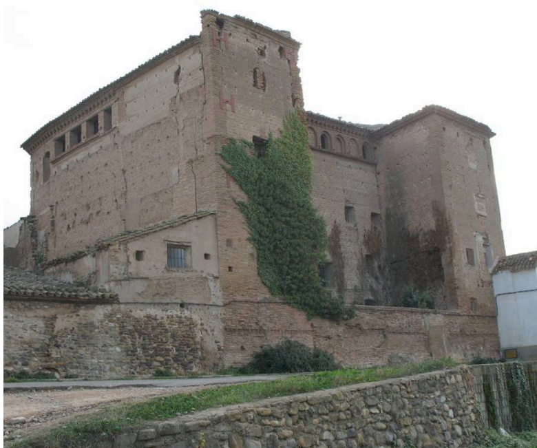
Fig. 1. The preceptory at Ambel, north-east elevation. The gallery of arches between the towers is typical of 16th century architecture in this region. The first phase precinct wall reaches the base of ivy and stands 3m high.
