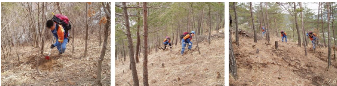
Figure 1 - Fire break line establishment methods (a: group of one, b: group of two, c: group of three)
