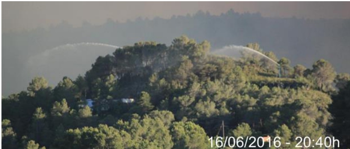
Figure 5 - Image taken on 06/16/2016 at 8:40 p.m. from Barraca d'Aigües Vives. It shows WUI-PROTECT® monitors of sector 3 providing water to the perimeter before the arrival of the flame front. Source: Vicent Vila.
