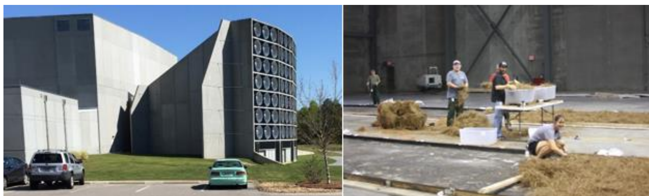
Figure 1 - Exterior photo of IBHS facility with fans (left image) and experimental chamber (right image) where staff are constructing fuel beds in preparation for a burn.
