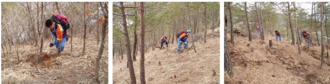
Figure 1 - Fire break line establishment methods (a: group of one, b: group of two, c: group of three)
