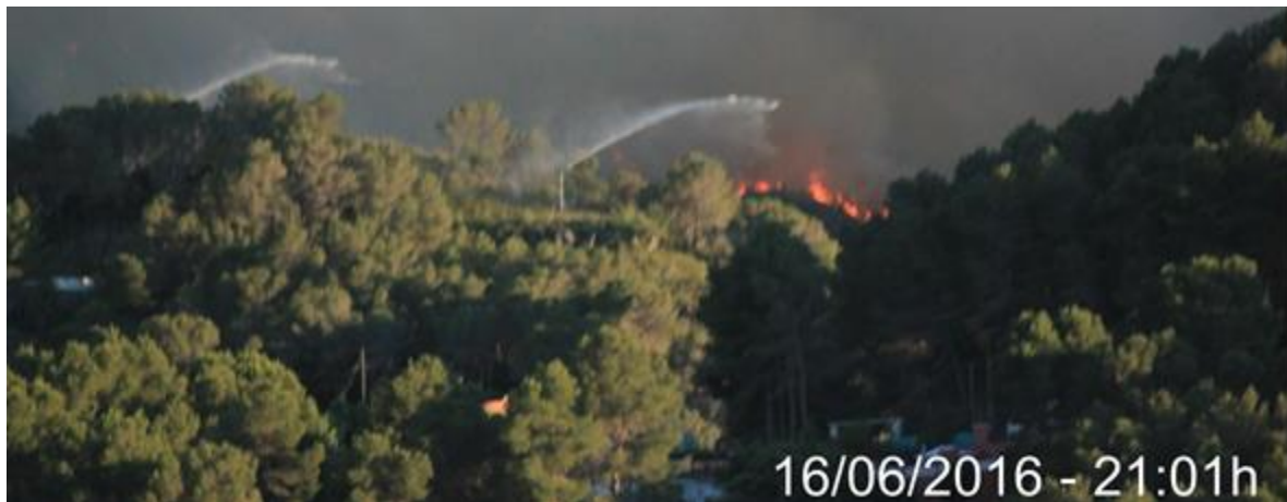
Figure 6 - Picture taken at 9:01 p.m. from Barraca d'Aigües Vives. It shows WUI-PROTECT® monitors of sector 3 as they continue supplying water, in this case outwards, before the arrival of the flame front. It shows that the water reach is less outwards due to strong upwind. However, this effect was offset with a bigger water inner scope. More water inside and less water outside. Source: Vicent Vila
