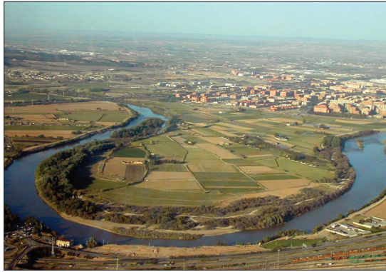
Photo 7 - The Meandro de Ranillas before the interventions; in the background, Zaragoza’s Actur neighbourhood (Source: Alday et al., 2008b).
