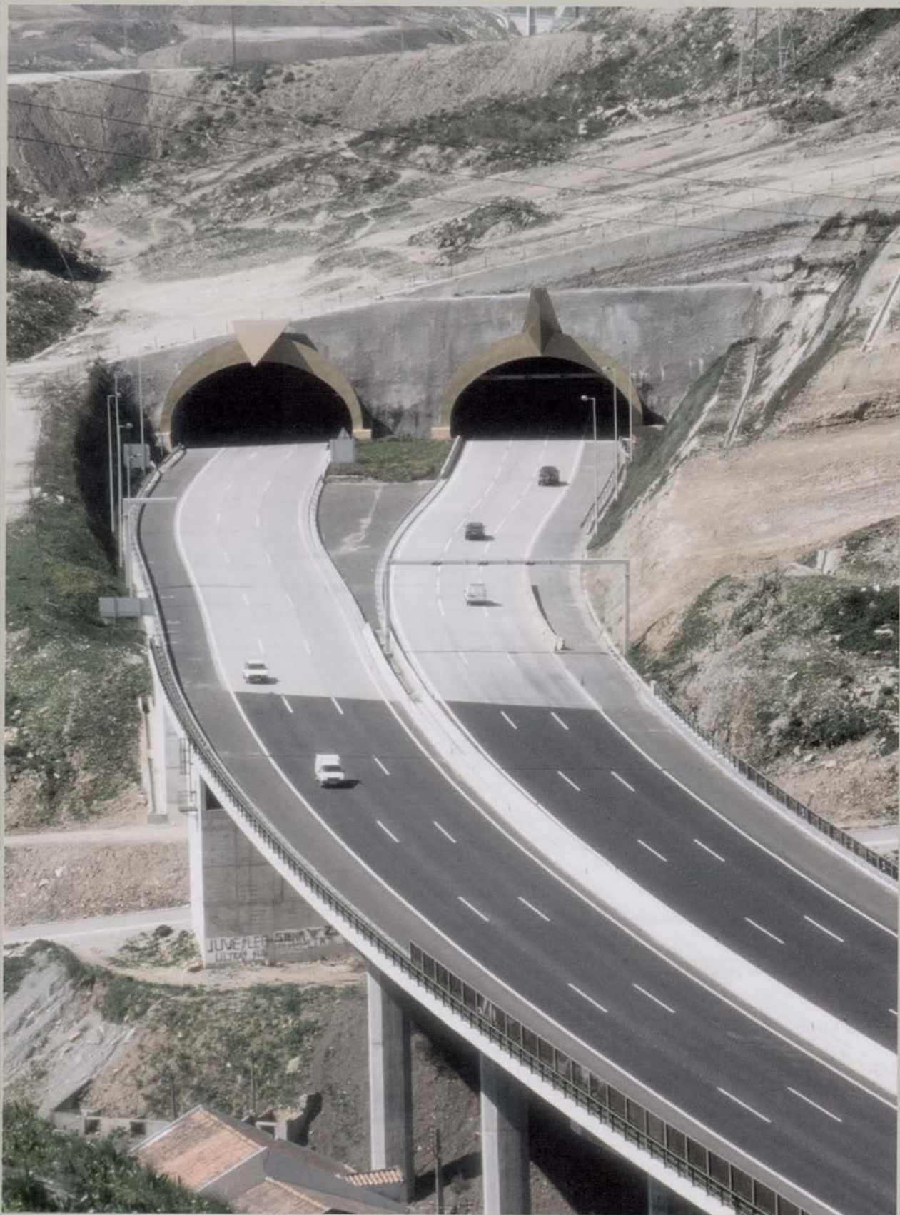
Vista lado norte, transição das galerias dos túneis com as pistas rodoviárias View of north side, transition from tunnel galleries to roads
