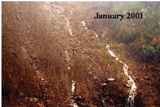
Photo 10 – Location of the occurrence of the debris flow of Volta Grande which affected road N101 and dragged two cars causing one death among the car occupants.
