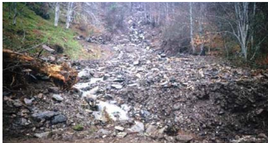
Photo 7 - Another detail of the debris flow in Póvoa da Serra.
