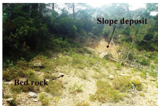
Photo 8 - Detail of the place where the debris flow of Portal da Freita began, whose failure is clearly related with the contact of the deposit with the bedrock.
