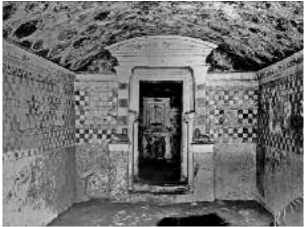
Fig. 4: Anfushi II . The Upper landing of the stairs.
