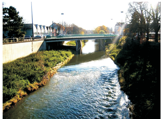
Photo 1 - The diversion canal of Ill in Mulhouse.
