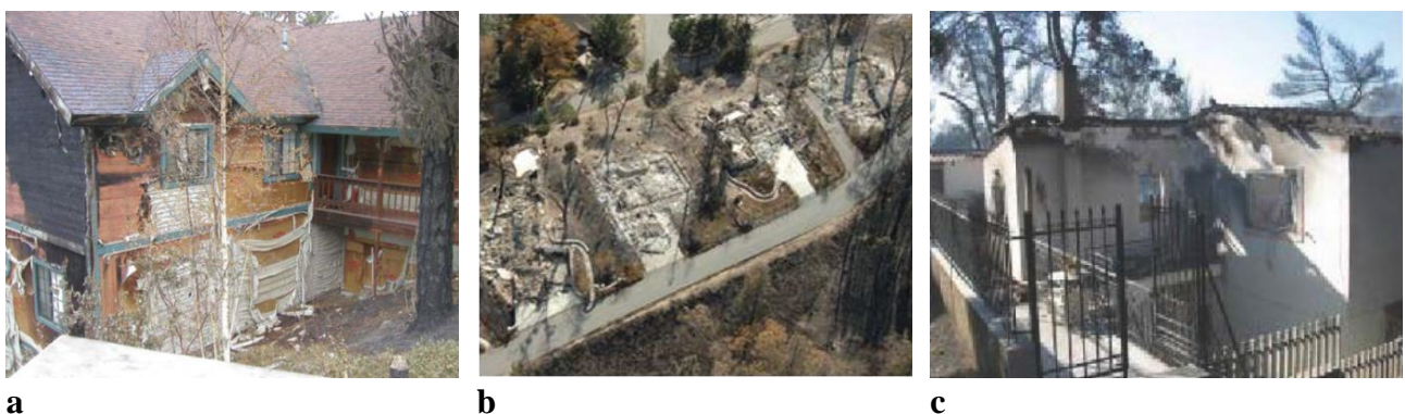
Figure 1. Influence of the construction materials characteristics on building vulnerabilities to wildland fire threats: a) building envelope damage due to the combustible construction materials (U.S.A.) (Cohen and Stratton, 2008); b) buildings destruction due to house-to-house fire spread (U.S.A.) (Cohen and Stratton, 2008); and c) building destruction due to its combustible contents (Greece) (Xanthopoulos et al. , 2011).
