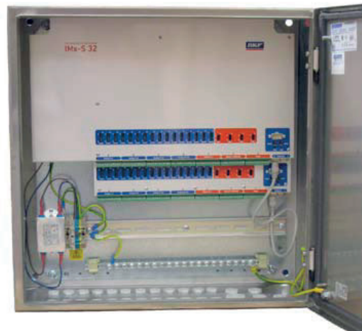
Fig. 4 - System SKF IMx'S
