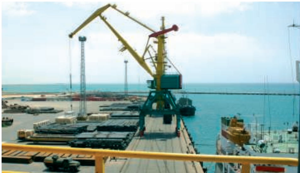
Kazakhstan, Traceca, renovation of Aktau ferry terminal © EC/Ruslan Alekseevich
